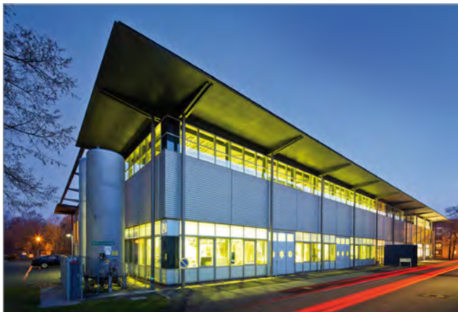
Technical center building of Fraunhofer FEP with efficient heat pump concept
