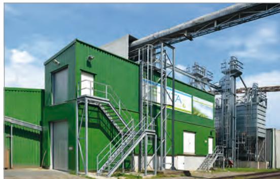
Exterior of the first E-VITA system in Güstrow, Germany
