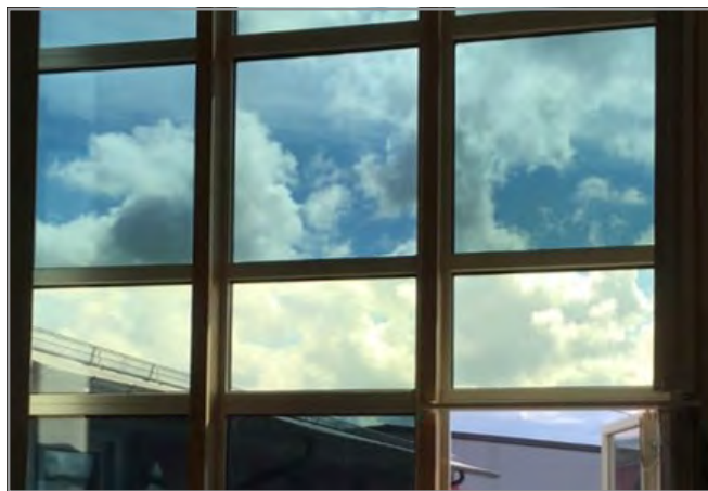
Figure 1: Visual comparison between electrochromic windows in non-switched (bottom) and switched (top) state.
